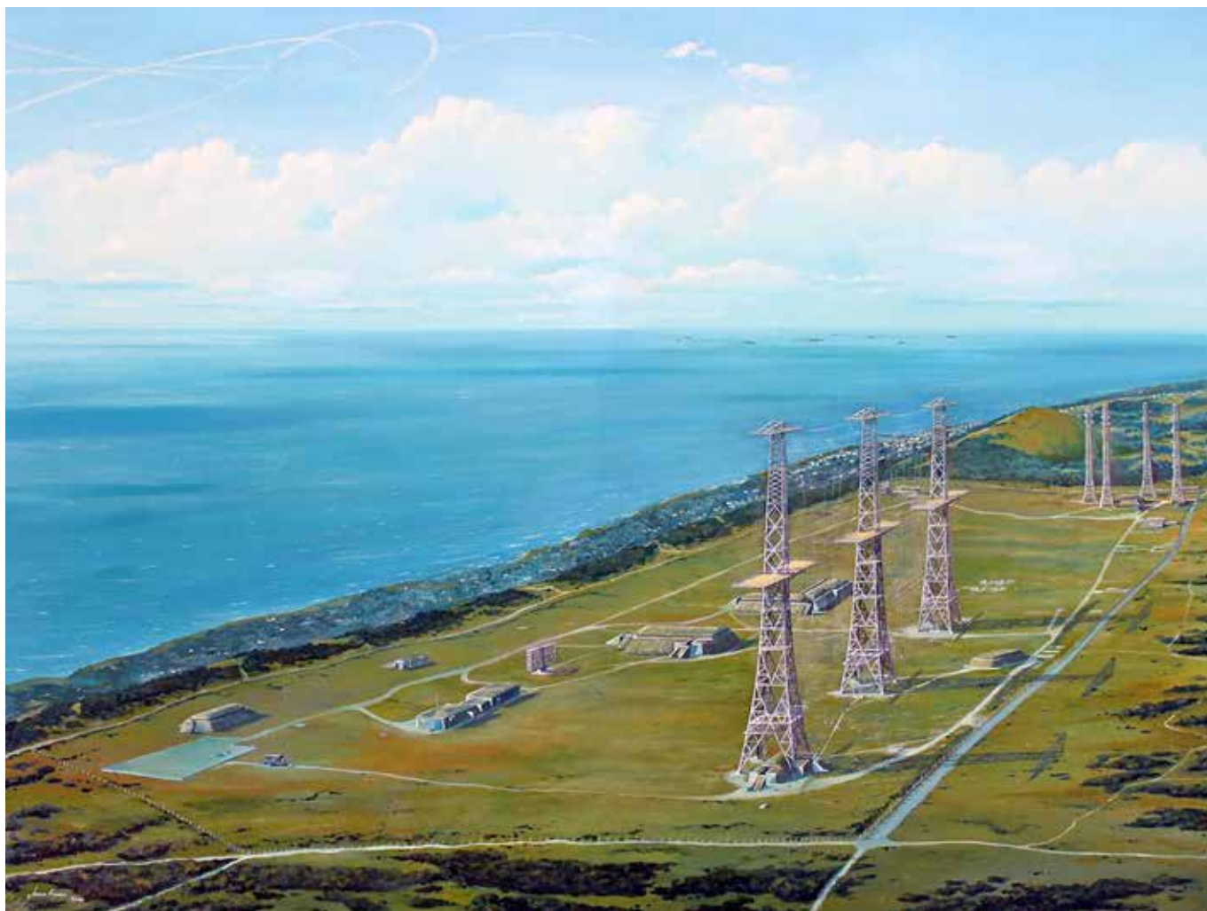
RAF Ventnor – three steel transmitter towers in the foreground and four timber receiver towers in the background.
